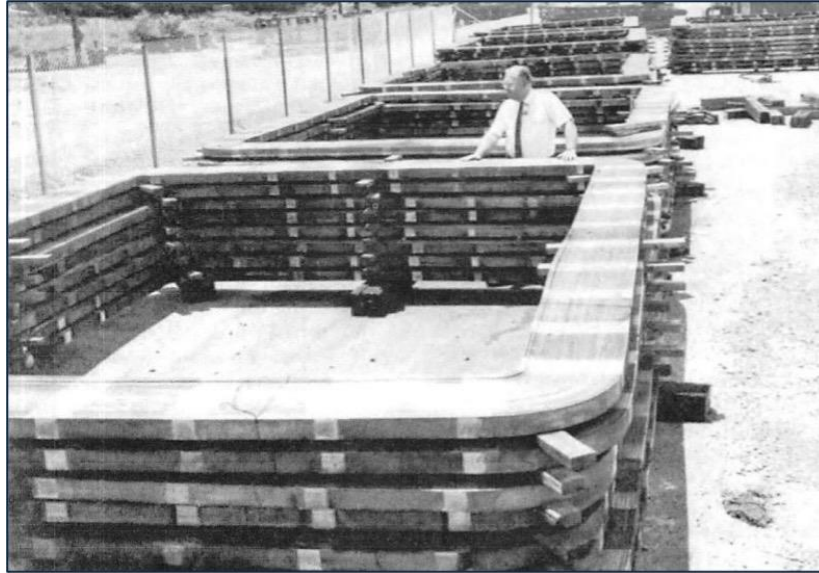
Silver-wound Magnet Coils for the Electromagnetic Process (Photo by Ed Westcott)
